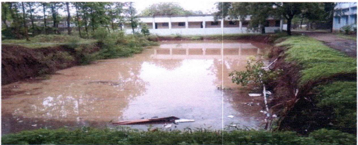
Check Dam Constructed in the campus
